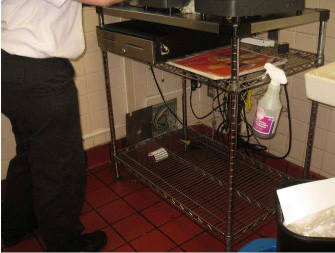
Most likely Point of Conduit entry
